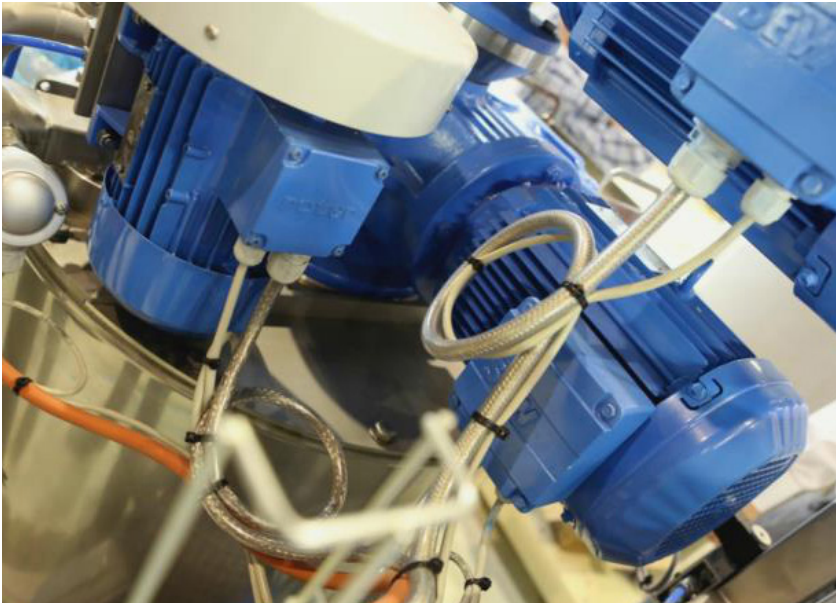
Loops along the cables trap dirt and are tough to clean and therefore should be avoided in food production.
