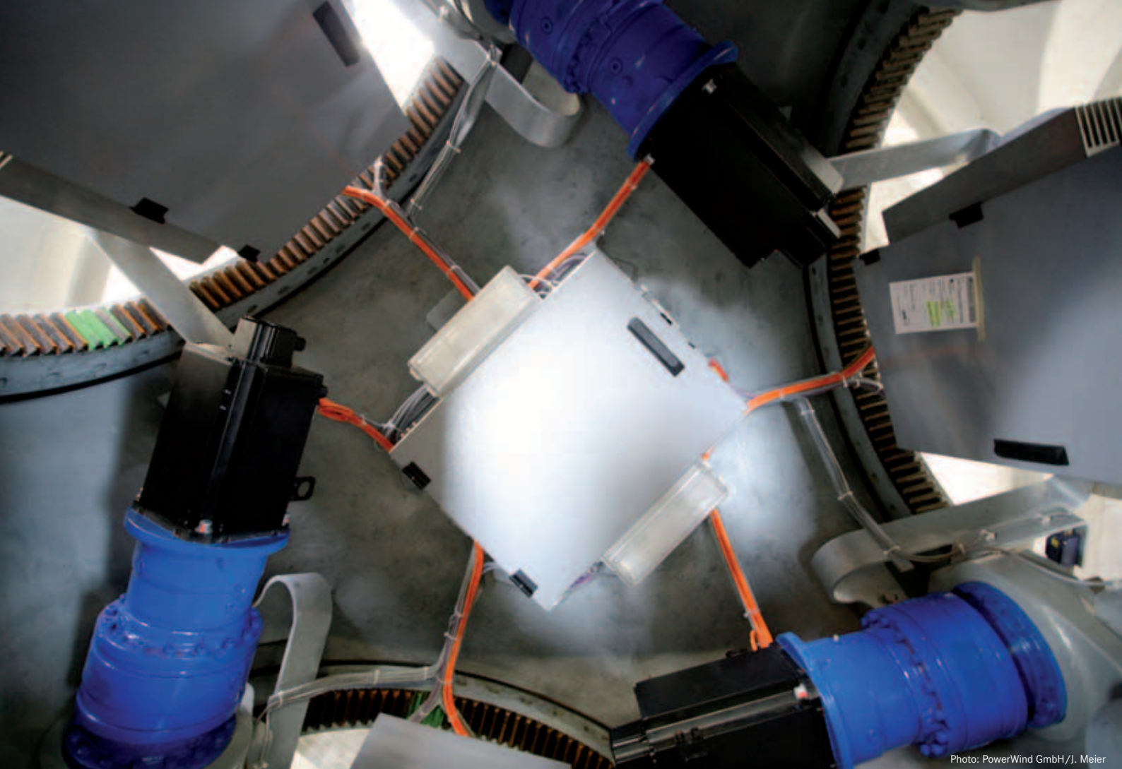
Photo: PowerWind GmbH/J. Meier
