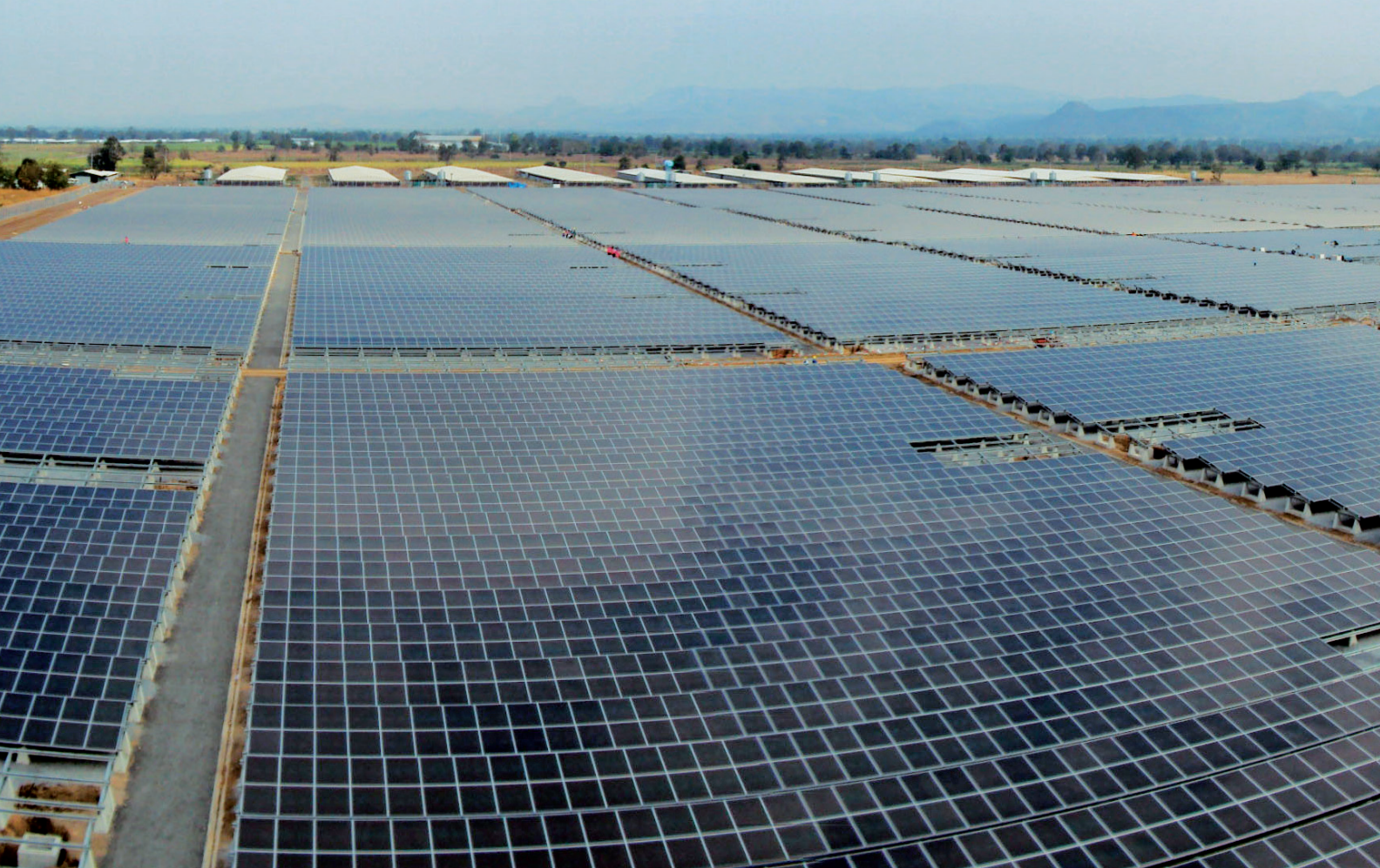
One of the world's largest photovoltaic power plants is being installed in the Lop Buri province, Thailand. – The connections are made using ÖLFLEX® SOLAR by Lapp
