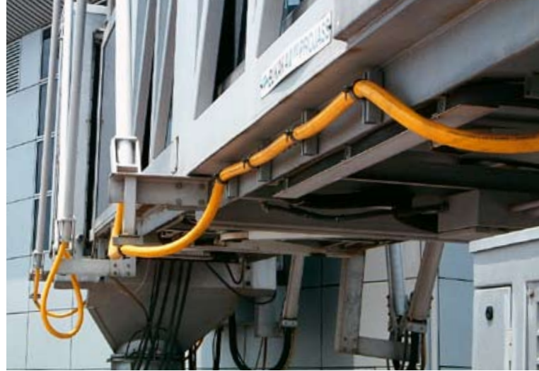
Kuala Lumpur International Airport, BETAjet® 400 FRNC-smartflex-V cable
