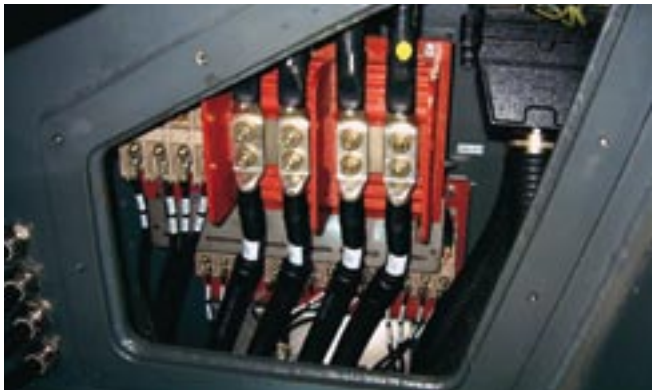
Panels, Cubicles and Systems
