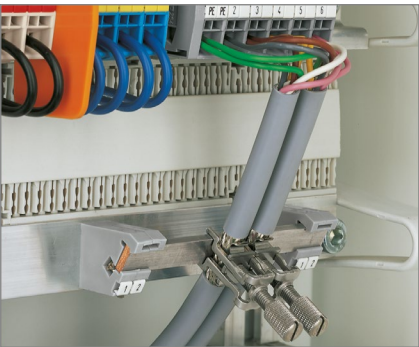
Insulated mounting carriers for a common shield reference potential, independent of housing potential ④ ⑤ ⑥ ⑦ 14 15 16 28 29
