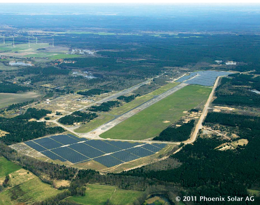
Aerial view of Preschen Solar Park
