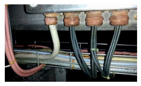
In the food and beverage industry, cables and cabling components are subjected to particularly strenuous conditions. If unsuitable components are used, then screw joints could corrode and the cable insulation could swell, as can be seen in the image. The components would lose some of their functionality and it could result in hazardous situations.
