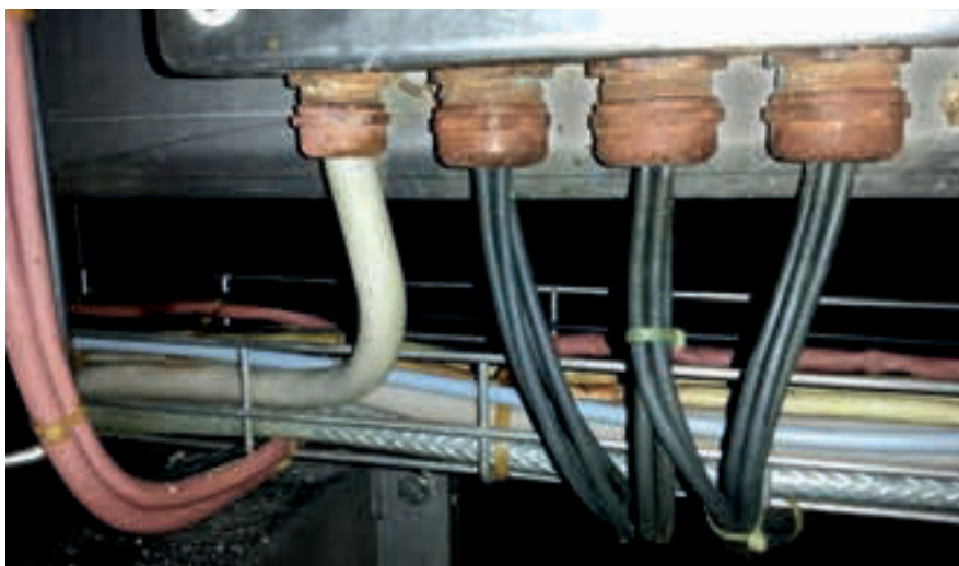
In the food and beverage industry, cables and cabling components are subjected to particularly strenuous conditions. If unsuitable components are used, then screw joints could corrode and the cable insulation could swell, as can be seen in the image. The components would lose some of their functionality and it could result in hazardous situations.
