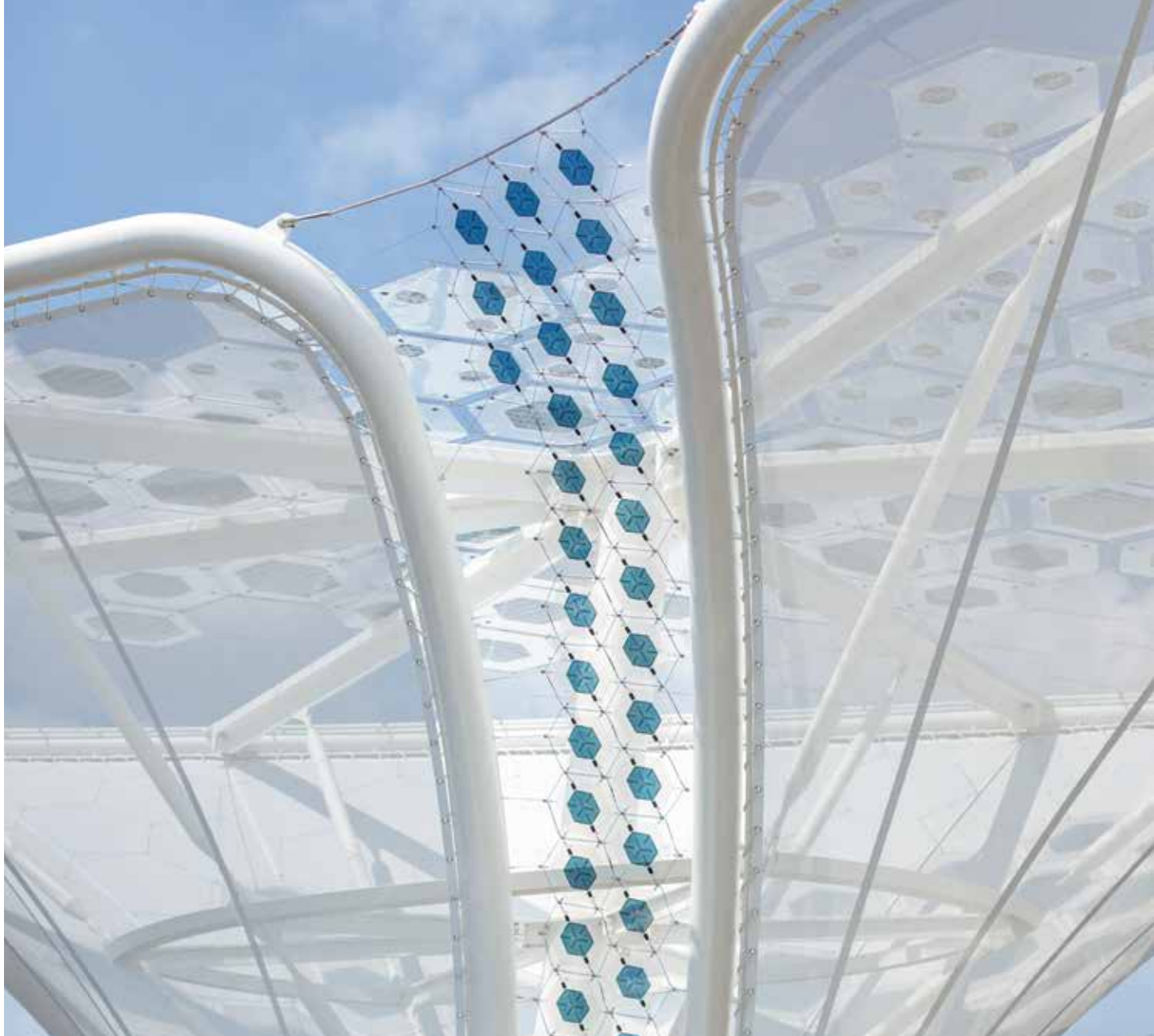
Organic photovoltaic objects on German pavilion at the world exhibition in Milan
