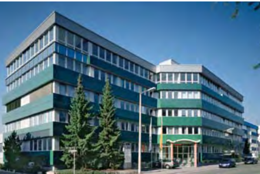
Lapp-Center in Stuttgart
