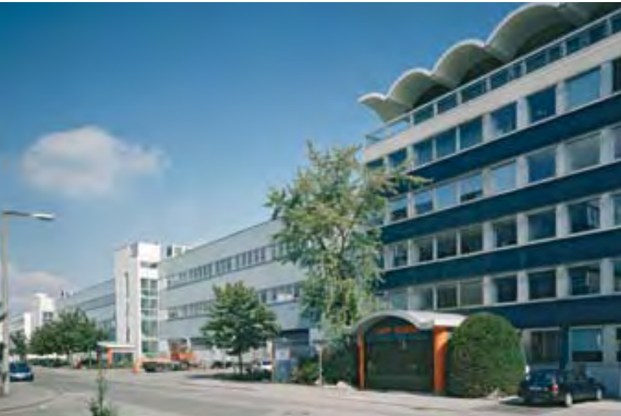
Headquarters in Stuttgart
