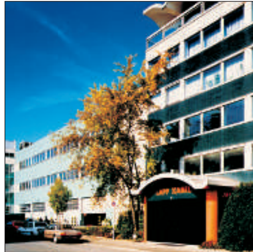
The Lapp Kabel headquarter in Stuttgart-Vaihingen.
