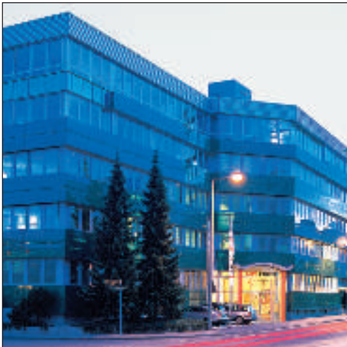
The Lapp Center in Stuttgart-Vaihingen
