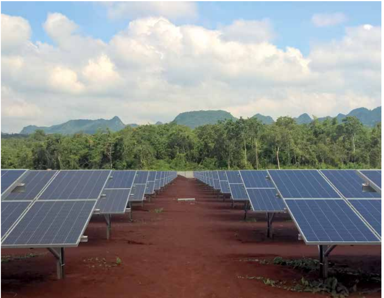
The 18 MWp solar unit in Kanchanaburi Province.
