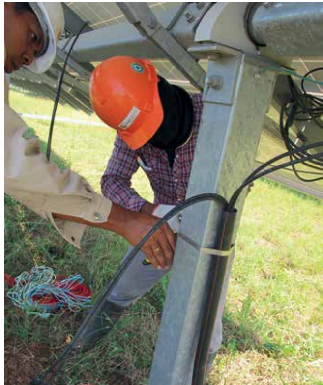
An employee installs the waterproof solar cable.
