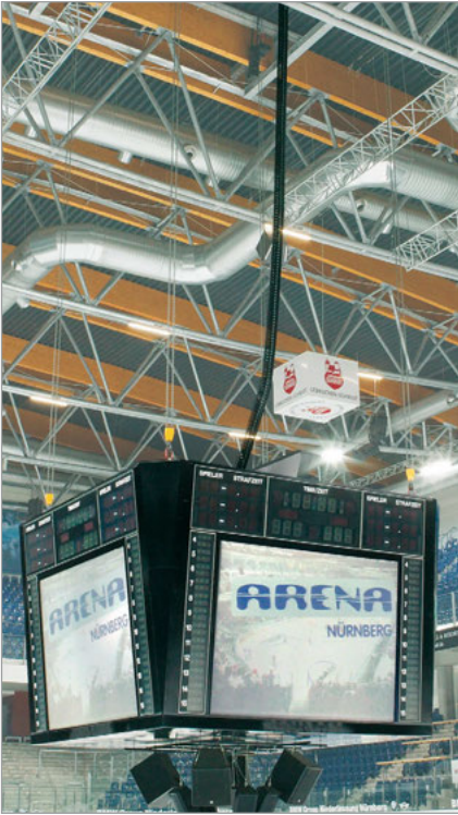
UNIFLEX cable carrier system in a zig-zag system on a lowerable multimedia cube in the Nuremberg Arena
