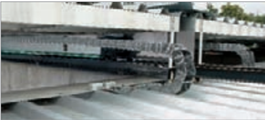
Steel cable carriers on a movable roof construction Photographs: Lindenschmidt KG
