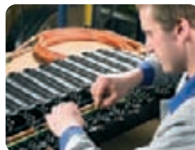
Complete assembly and commissioning with system guarantee
