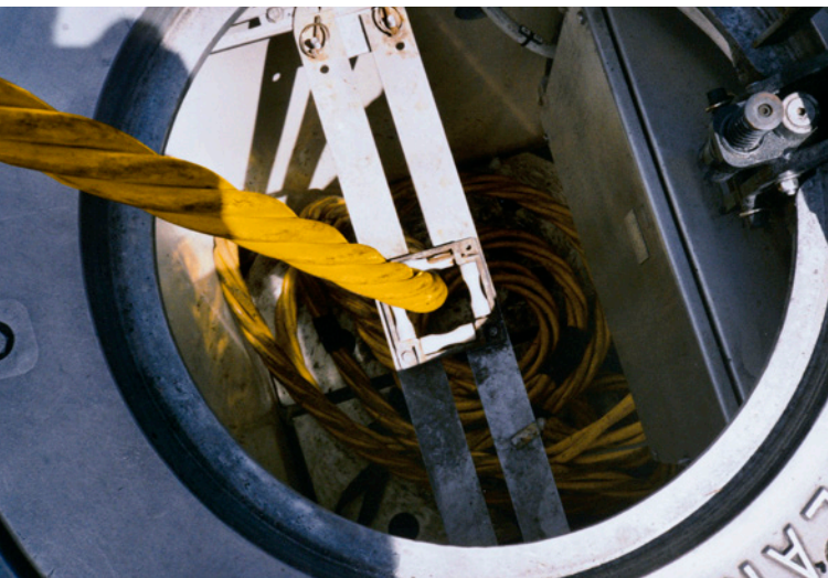
Zurich Airport, BETAjet® 400 FRNC-deltaflex cable
